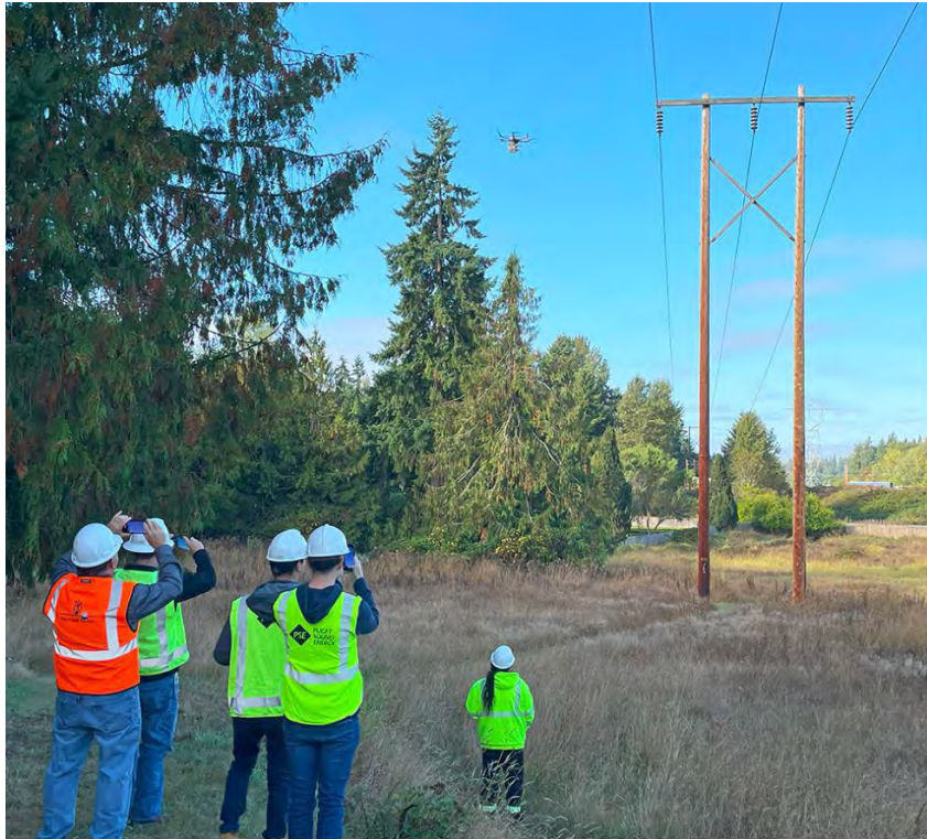
A drone installs the first DLR sensor on a transmission line in Pierce County, Sept. 2025.
