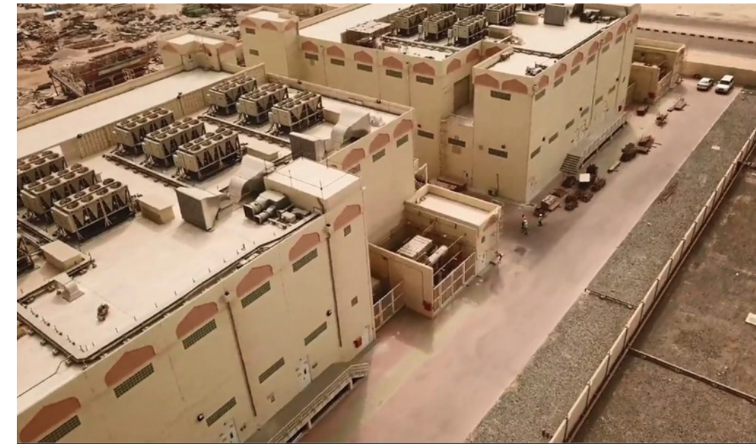
One of three NGK 20MW - 120 MWh NaS Batteries 108MW/648MWh installation in Abu Dhabi.
